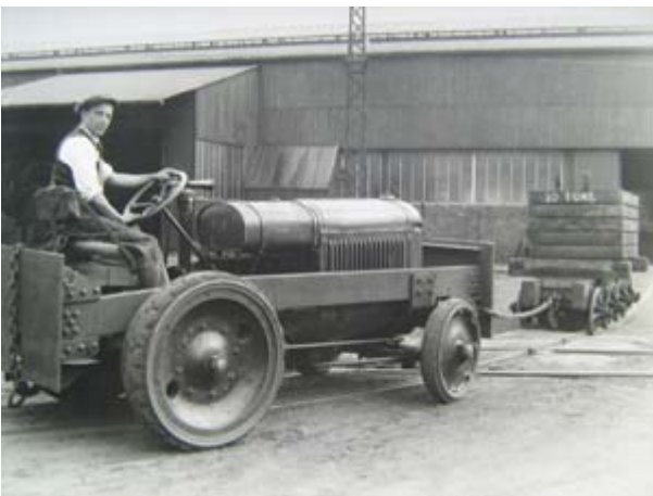
Primitive plateway at the Horsehay Works, which so surprised Rolt when he saw it still in use in the 1940s for building “D” Day barges. (IGMT. 1993.2254)
